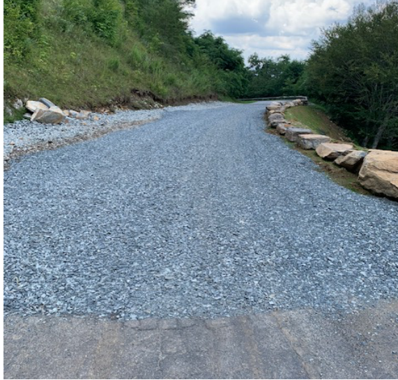
Photo: Buffalo Nvno repair complete
