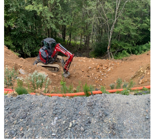
Photo: Buffalo Nvno repair in progress
