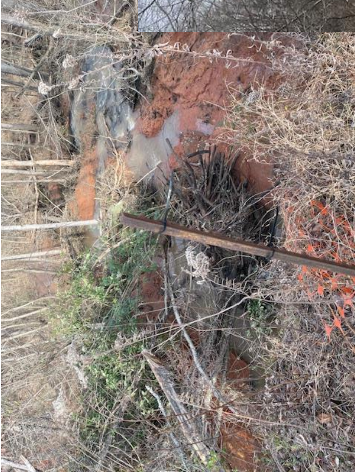
Additional erosion of the Dam and breach following Spring 2024 Rainstorms
